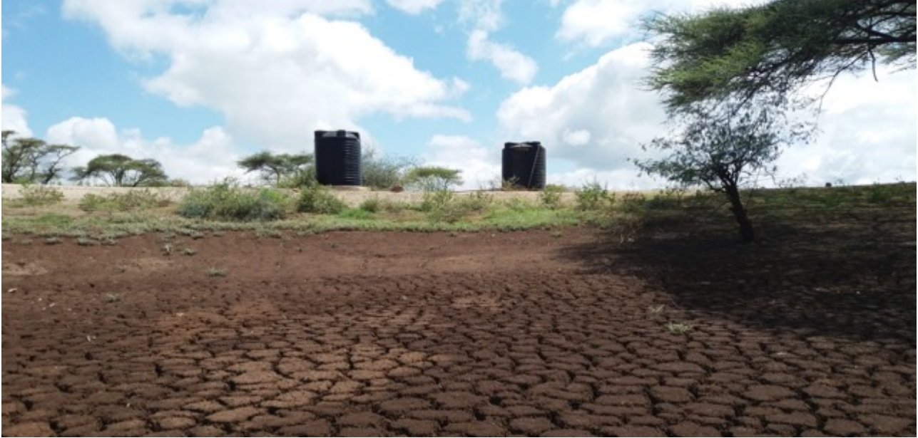
Water pan near Kinna, with storage tanks via which water is piped to taps and troughs.
