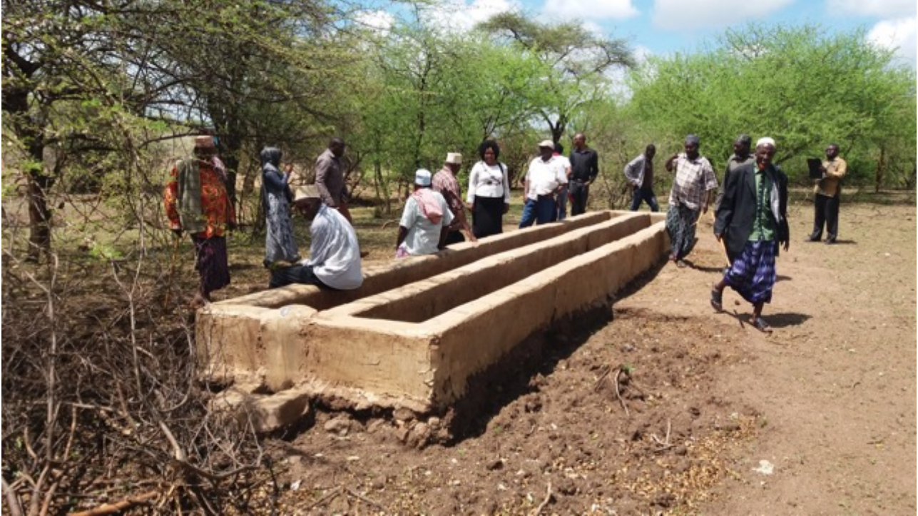
One of the troughs that receives piped water from the pan near Kinna, via storage tanks.
